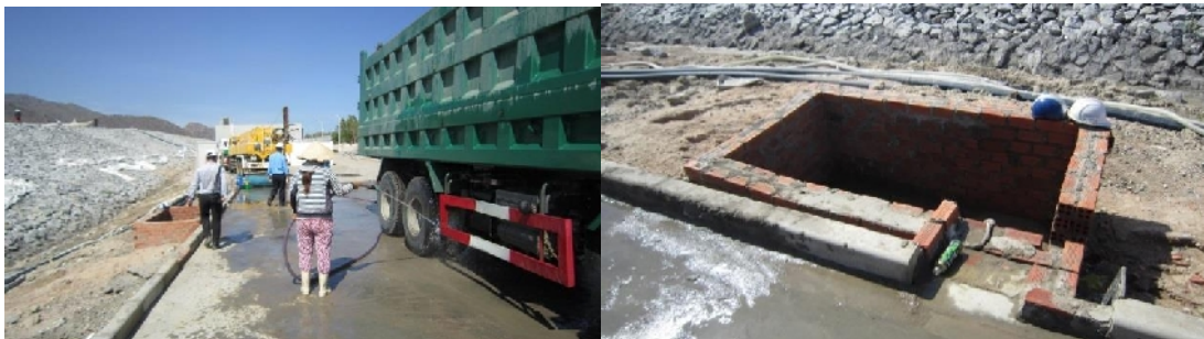
Figure 4.11. Washing down the trucks before leaving the ash pond and the waste water collecting pit
