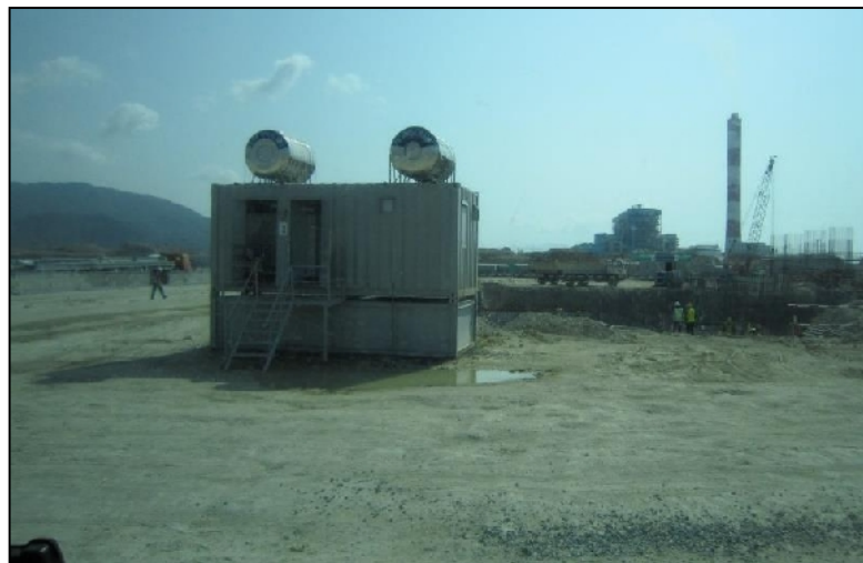
Figure 4.1. Mobile toilets in the construction site of Vinh Tan 4 TPP
