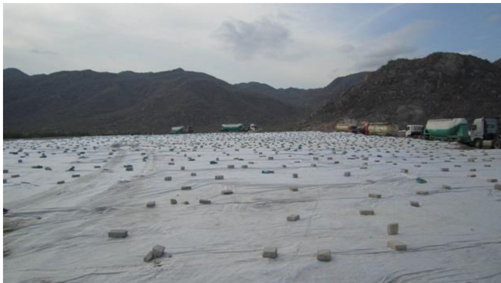
Figure 4.14. Watering and using tarpaulin to cover the ash pond surface at the bottom of Mount Ho Dua.
